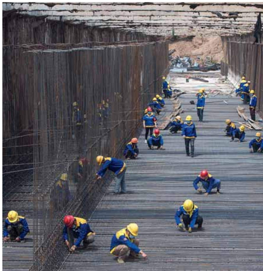
Construction workers in Wuhan, China, resume construction on a utility tunnel
